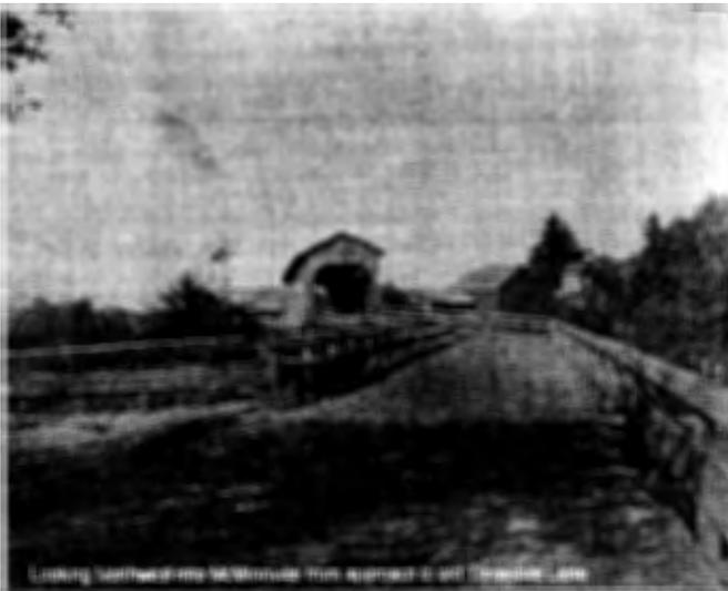
The completion of the Lafayette bridge was somewhat of a milestone in Oregon history. The cost alone set it apart from earlier territorial bridges, and it was a truss span, meaning that it was self-supporting, very unusual for the time. It would be ten years before any comparable span was constructed in the state. We may never know if this structure was of the covered variety, since details are very sketchy.
